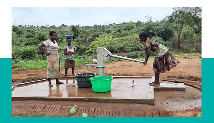
The project rehabilitated six water points providing communities with access to clean water, pumped through pipes drilled deep into the ground. Handpumps are fitted at each borehole meaning that water can be easily extracted for community use.
