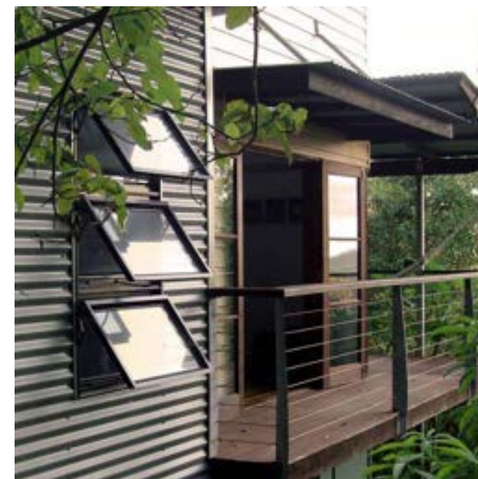
Image 39. Shaded openings and natural ventilation
