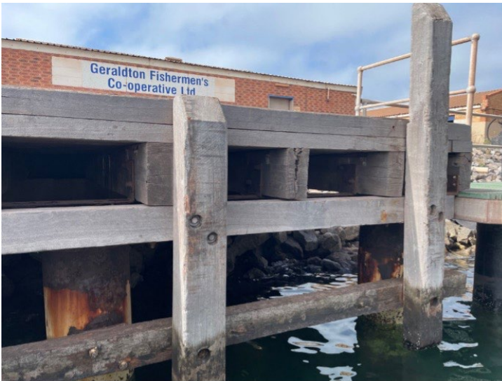
Figure 2: GFC Jetty; showing the low freeboard and physical obstructions; which presents challenges for access physical access and a clear line of sight for laser scanning
