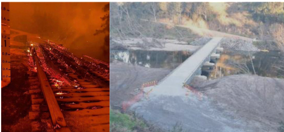
Figure 9. Left: Murphys bridge 31 December 2019 during the bushfires, Right: Murphy's Bridge concrete replacement, Source Eurobodalla Shire Council [14]
