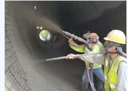
Shotcrete Pipeline Repair
