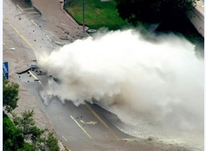
Los Angeles (USA) – Water Main Burst (2014)
