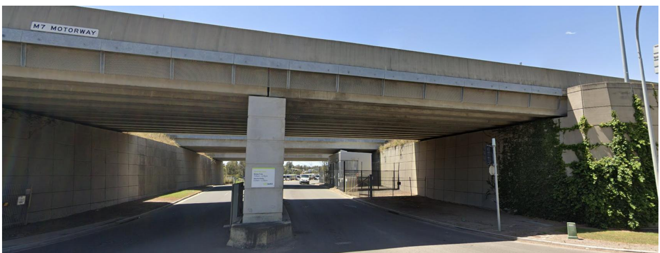
Figure 5. Bridges over the Waste Services Access Road Infra 25.10/25.11 – Switching Station.
