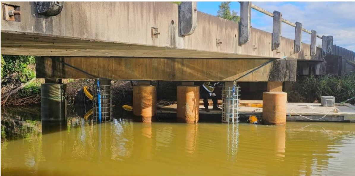
Figure 14. Pile encasement installation in progress
