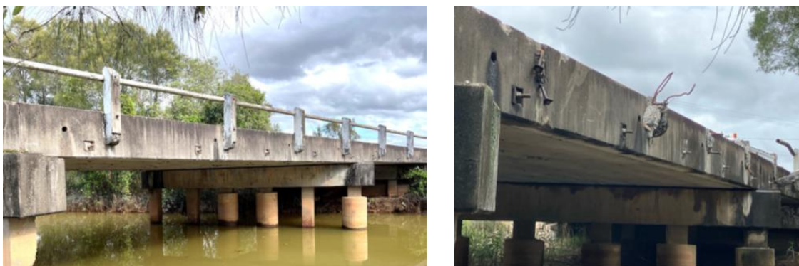
Figure 3. Left, Bridge barrier before the accident, Right, Bridge barrier
