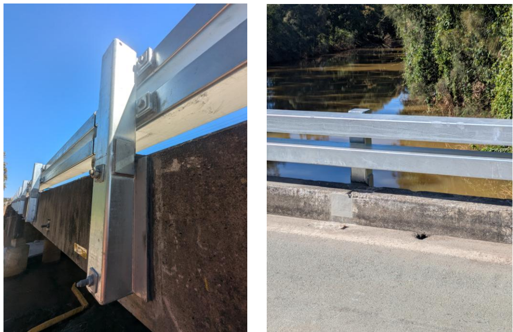
Figure 9. Installed bridge barrier
