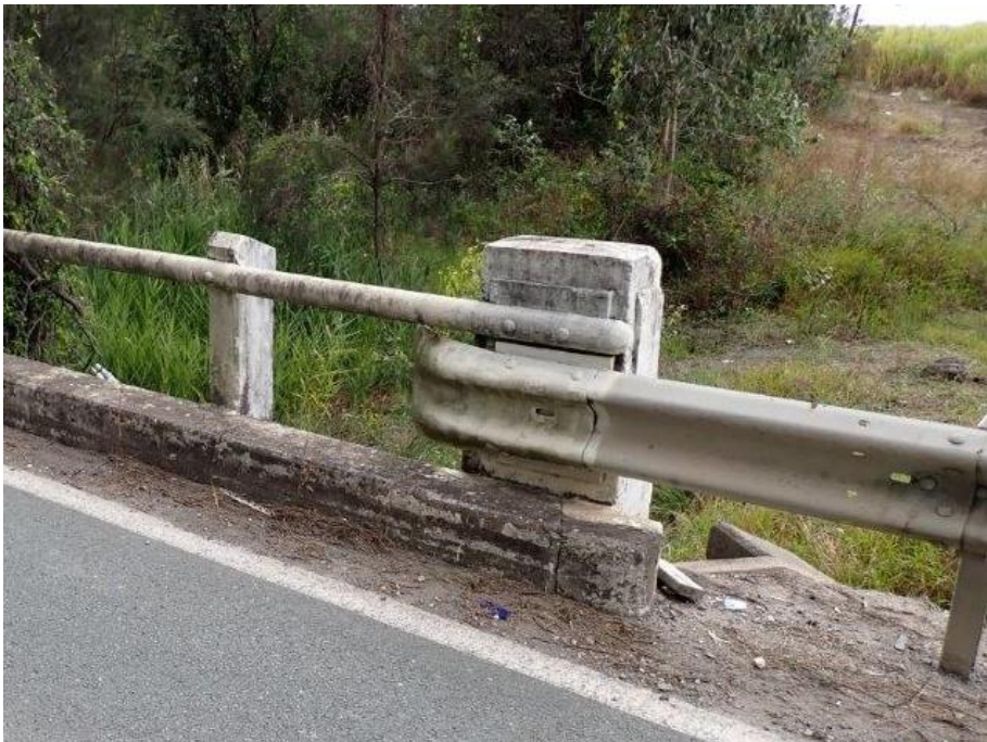
Figure 10. Typical existing approach barrier to bridge connection
