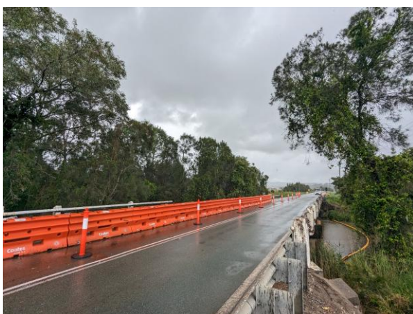
Figure 4. Temporary Traffic Control
