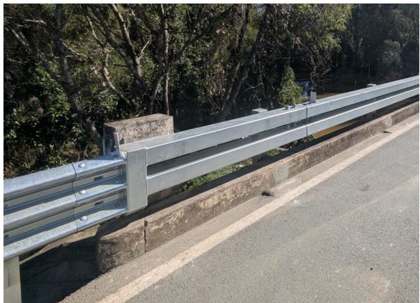
Figure 11. Installed guardrail transition in end post
