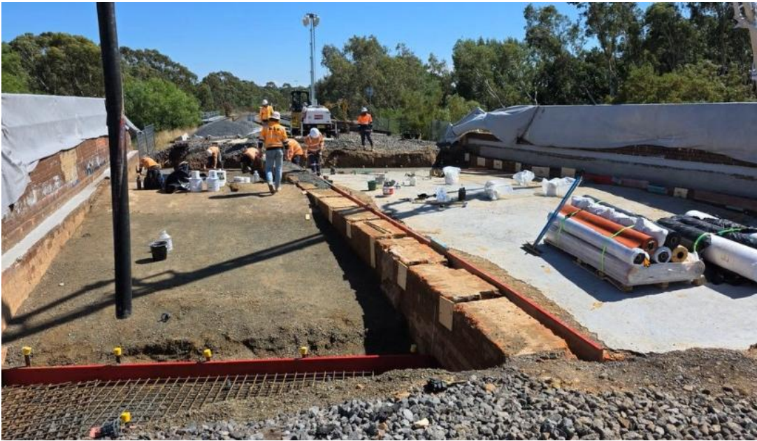
Figure 10. Waterproofing works – Looking down-track
