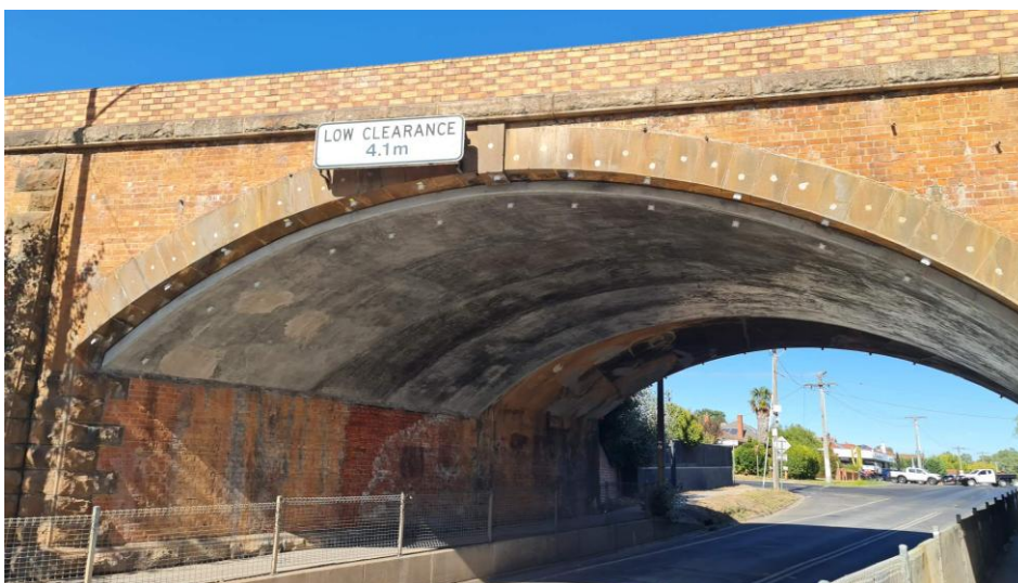
Figure 9. Completed soffit lining
