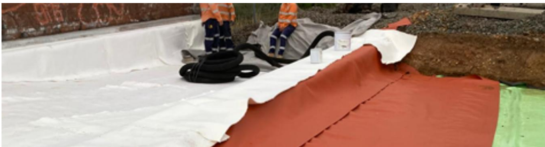
Figure 11. Waterproofing membrane and geofabric protection layer
